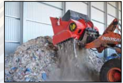
Crushing demolition waste
