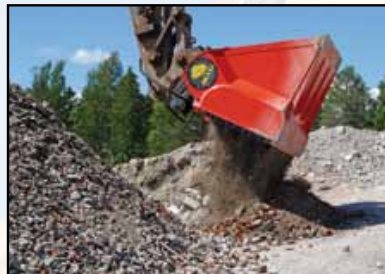
Crushing bricks / black top asphalt
