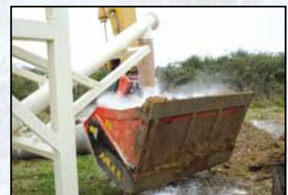
Stabilising soil with lime
