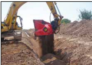
Pipeline padding/back filling
