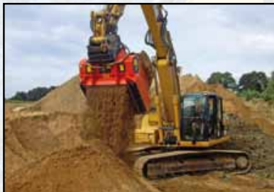
Mixing sand and clay
