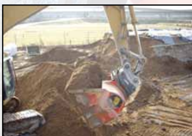
Stabilising foundation layers
