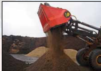
Mixing top soil and sand
